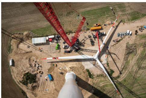
Assembly of wind turbines
